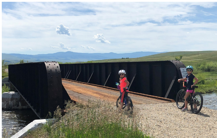
▲ Employee Family Members Take the First Ride on the Old Yellowstone Trail Project
