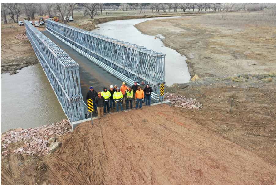
▲ EDA Funded Moorehead Bridge | Powder River County
