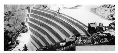
Basin Creek Dam #1 Shortly After Concrete Cap and Buttress Placement in 1913
