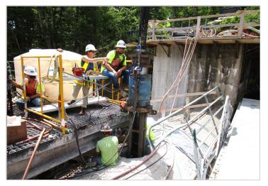
Crews Applying Post-Tensioning to Anchor
