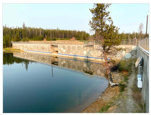
▲ Completed Dam Face Rehabilitation, Upstream Face of Dam
